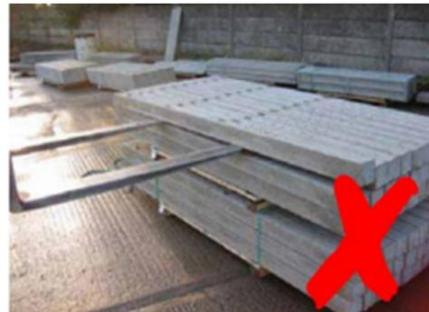
Products must not be taken out of packs using the forklift, they will damage the unit.
