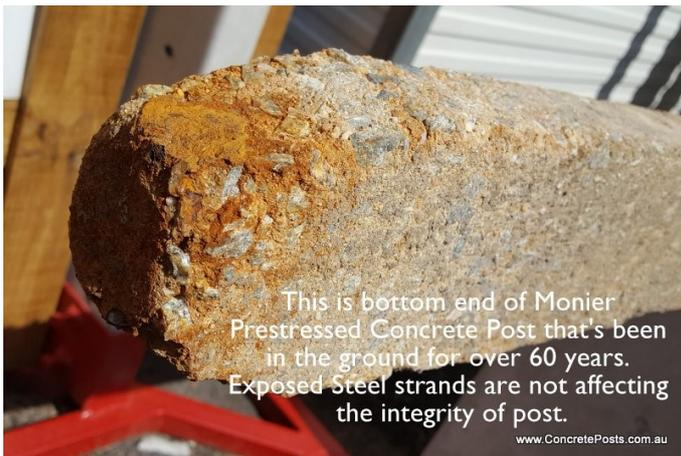
This is bottom end of Monier Prestressed Concrete Post that's been in the ground for over 60 years. Exposed Steel strands are not affecting the integrity of post.
