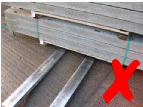
The forks must not be close together when picking up packs
